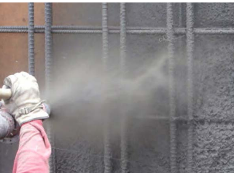
Fig. 1: Modern nozzle designs diffuse and accelerate the incoming mixture into thousands of individual particles moving within a high velocity nozzle stream.
