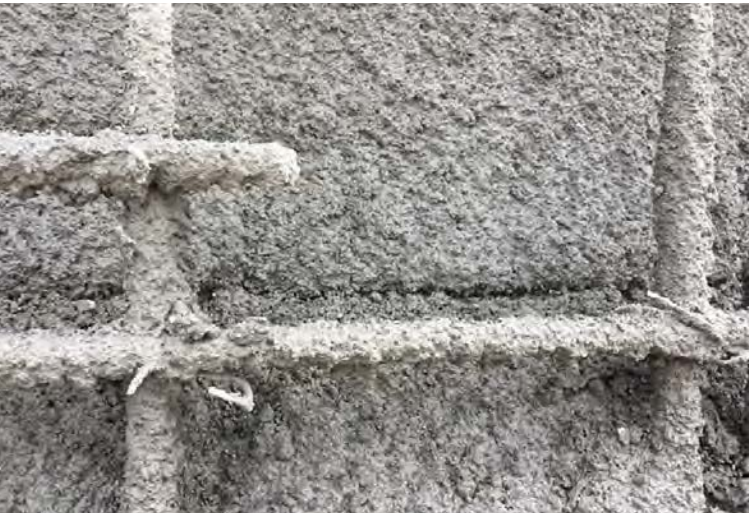
Fig. 6a. Tracking occurring within the shadow area is easy to see. Tracking behind reinforcements is visual evidence that the mixture is far too stiff.
