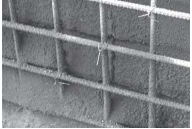
Fig.8. Freshly applied materials with a dull, rocky, or sandy surface is evidence of a mixture that is too stiff.
