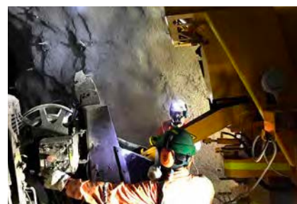
Fig. 1 & 2: Mixkret 6 during tests at the Chuquicamata mine, Chile
