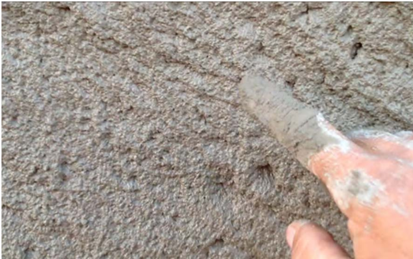
Fig. 9. Freshly applied materials with few visible aggregates at the surface is the visual indicator of a well-chosen slump.
